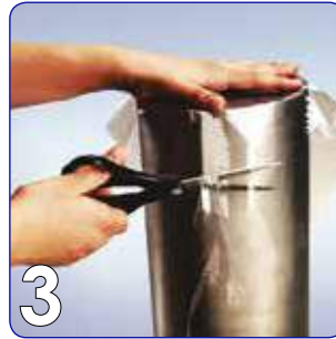
3 Cut LiquiFilm™ in a circle 1.3 times greater than pipe diameter
